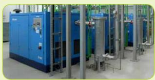
Oil-free and silicone-free compressed air generation is standard at BMW's car body manufacturing plants in Dingolfing in Germany.
